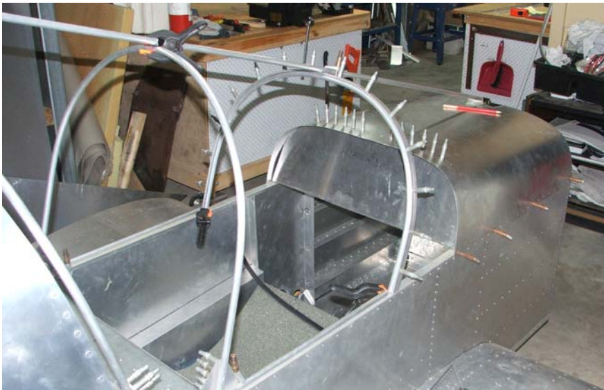
Instrument Panel and Coaming plus Canopy Framework under construction. A 55 Litre fuel tank will be positioned between the Instrument Panel and Firewall.
